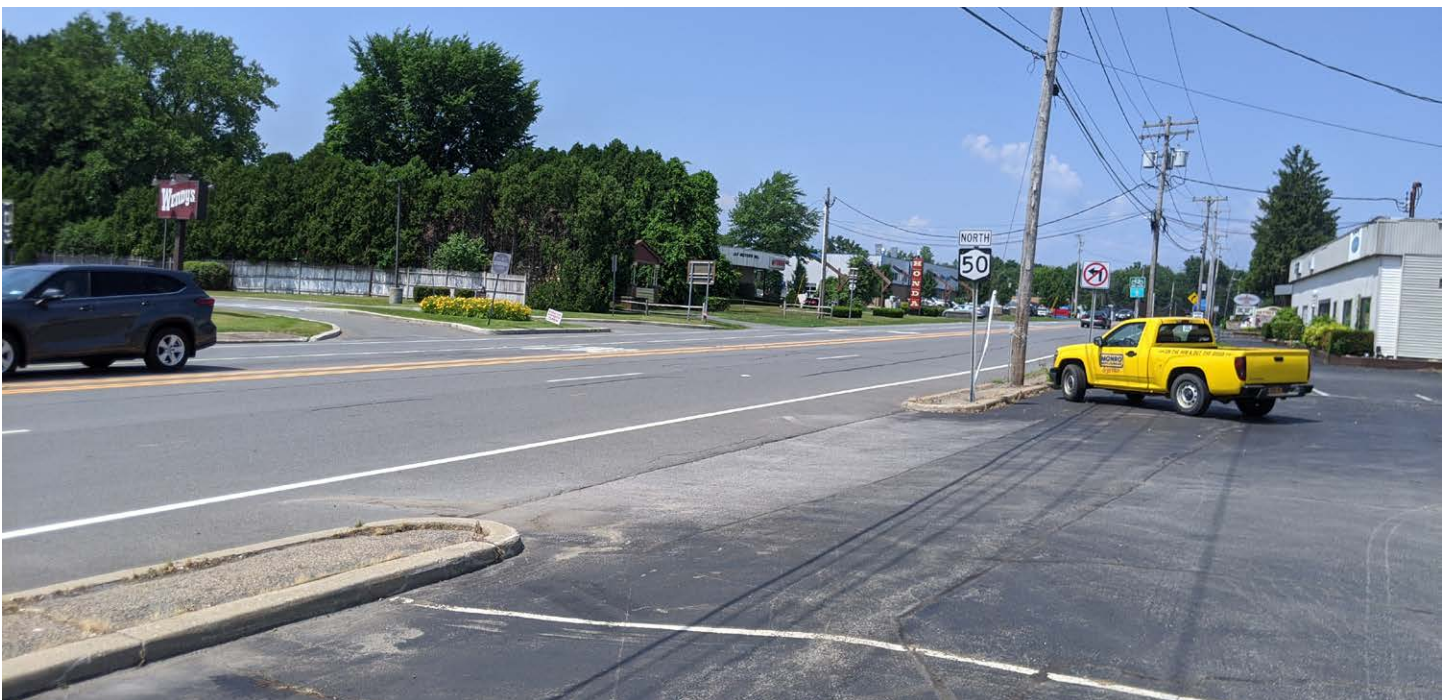
Figure 15. View looking north along Route 50 from Freemans Bridge Road. This section of the road is difficult to implement a safe pedestrian and bicycle route due to the high number of curb-cuts and vehicle turning movements.
