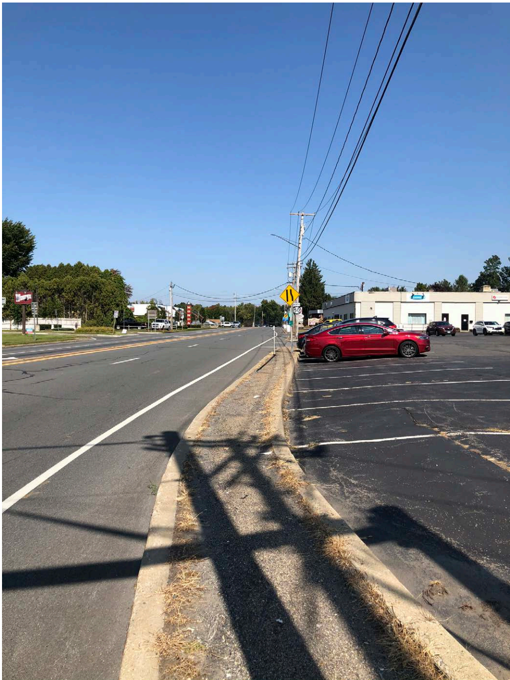
Figure 37. View along Route 50 looking north. The first ~1,500 feet along Route 50 from Freemans Bridge Road presents design difficulties and obstacles with narrow design widths and multiple curbcuts.
