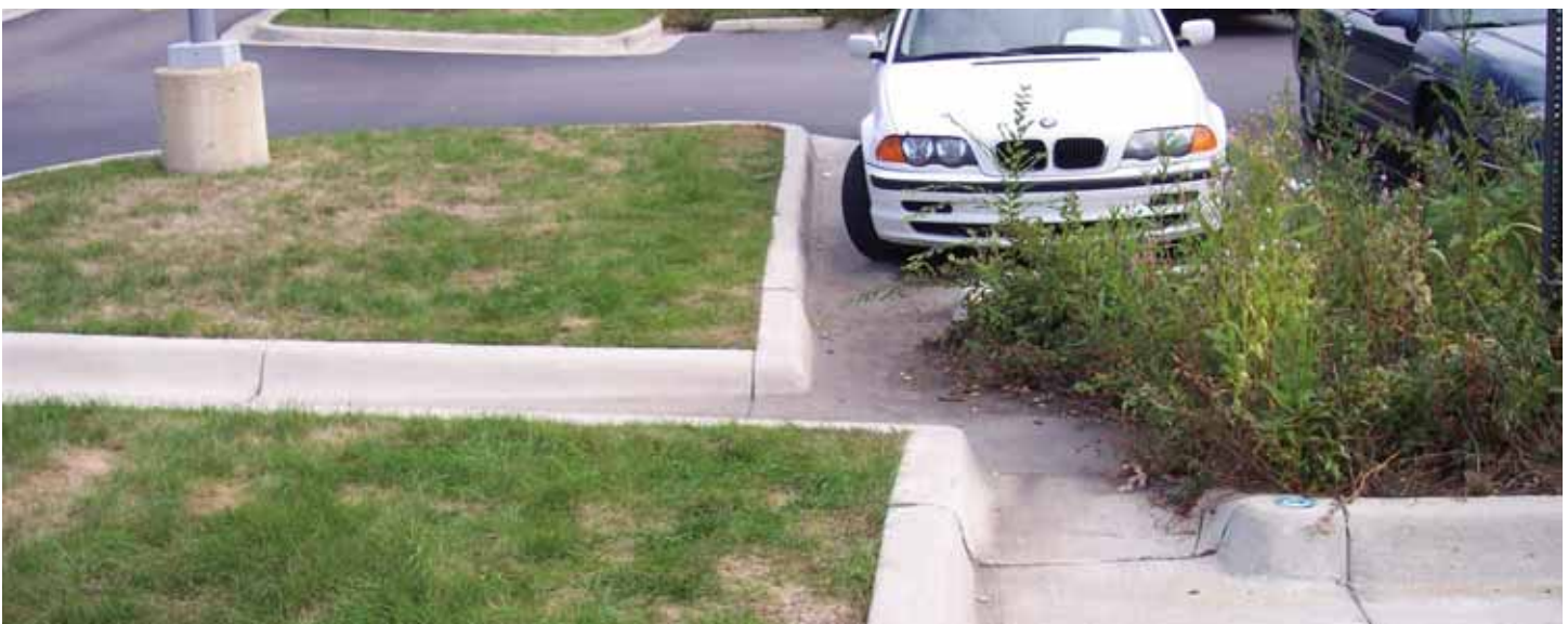
Simple techniques like breaks in islands allow for drainage to access areas more viable for Green Infrastructure installation.
