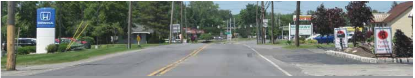
Looking north on Freemans Bridge Road - there are many open curb cuts with little definition and utility poles close to the road.
