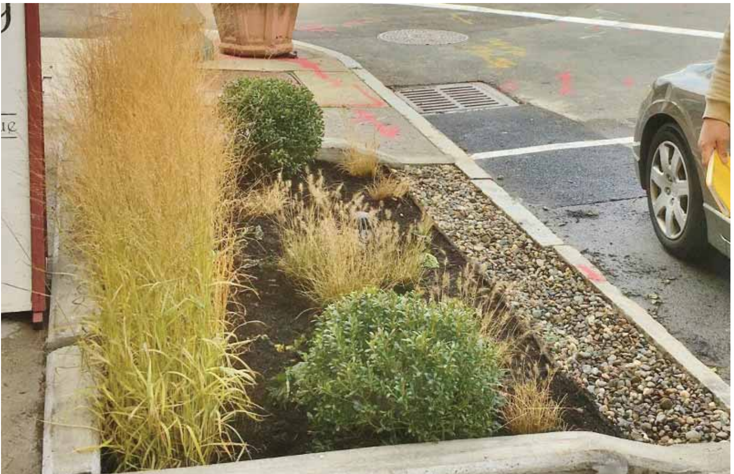
Green Infrastructure planters can be placed in areas with space constraints. (Photo courtesy of CDRPC)
