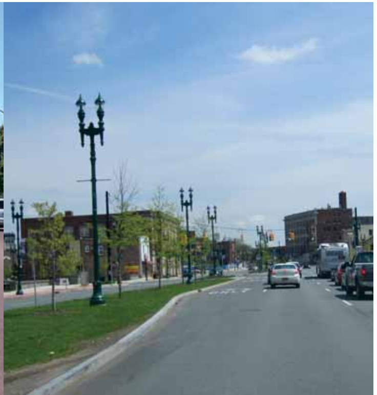
Example of a low, planted wide median in Schenectady, NY.
