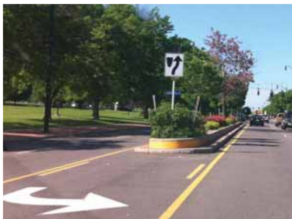
Example of a raised median on a 4-lane roadway in Buffalo, NY.
