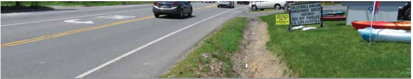
Looking north on Freemans Bridge Road - an open ditch with no green infrastructure or stormwater management elements.
