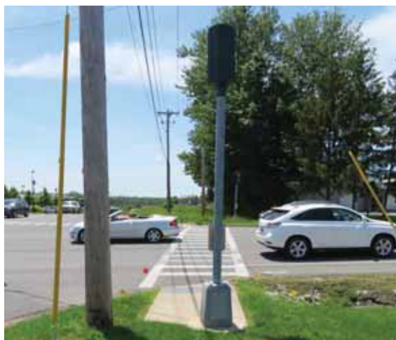
Sidewalk segment with crosswalk and pedestrian signal...though placed in the sidewalk
