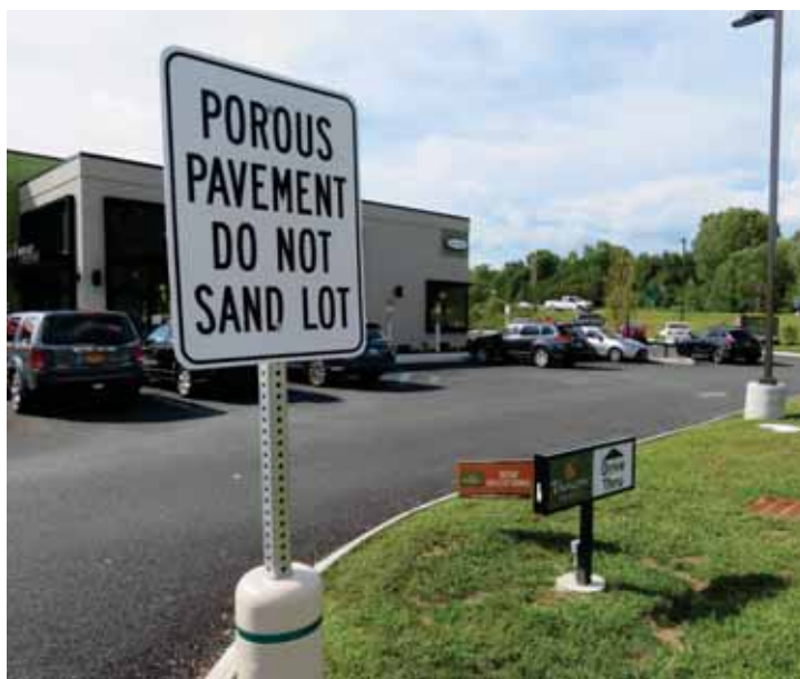
Examples of porous parking lots: This one is in Malta, NY.
