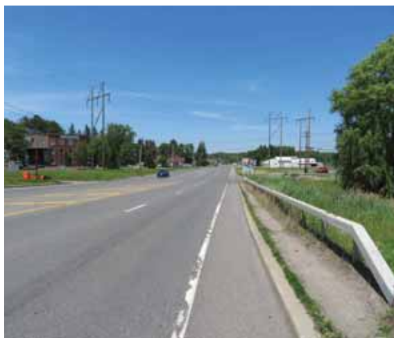
4-lane cross section with center turn lane just north of Freemans Bridge
