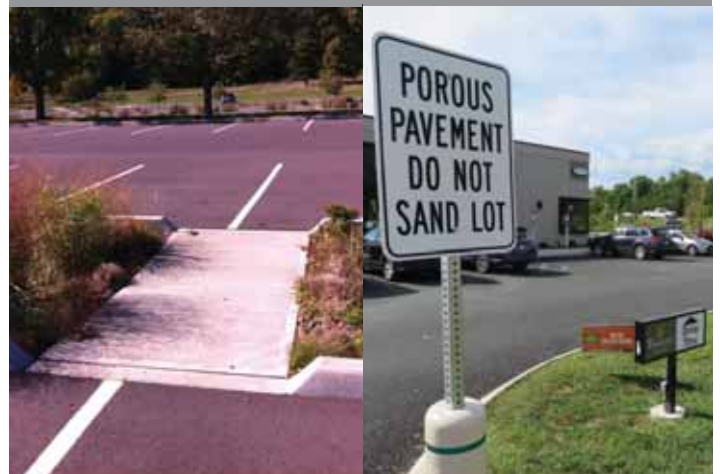
Sidewalk integrated into stormwater capture area of a parking island.
