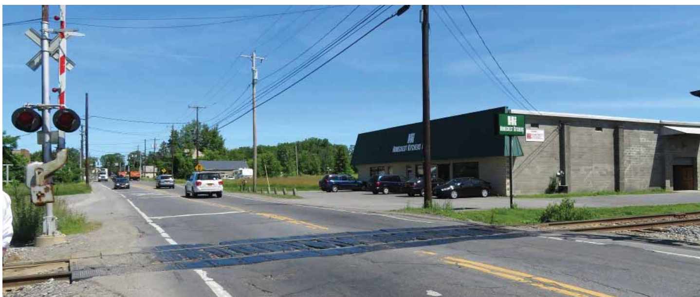
Freemans Bridge Road Railroad Crossing - this crossing is in bad shape and is scheduled to be upgraded in the near future.
