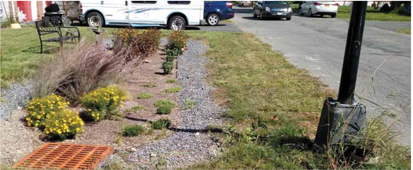
Vegetated non-curbed swale located along Marietta Place in Albany, NY. (Photo Courtesy of CDRPC)
