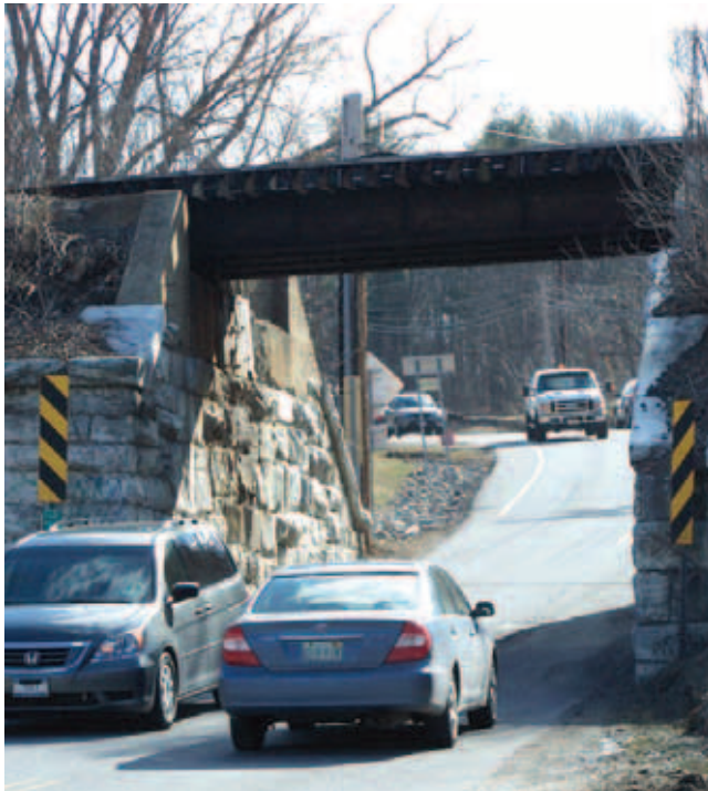
Pictured above: One of the two Glenridge Road overpasses to be replaced and widened.
